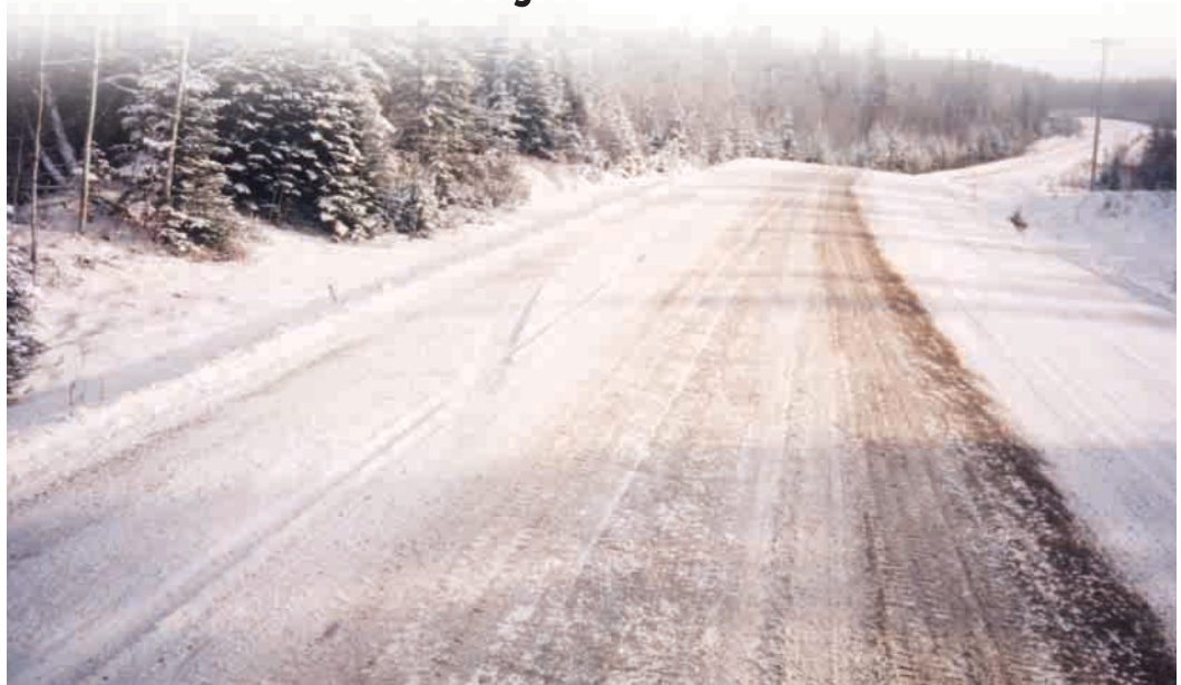
Pre-wet sand: one of the technologies MTO is testing to improve winter driving conditions.
